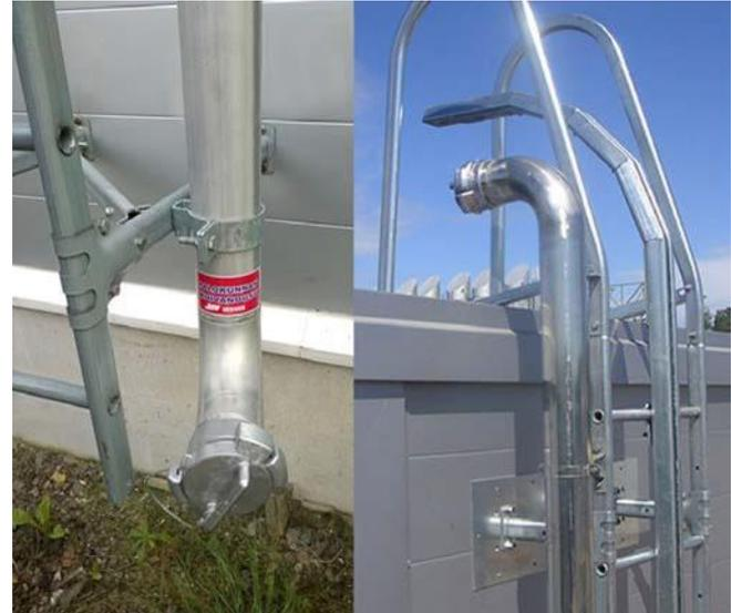
The dry riser pipes can be attached either directly to the wall or to the service ladder using additional support parts. The bottom and top of the pipe must be adequately supported. The lowest legs of the ladder are attached to the plinth.
