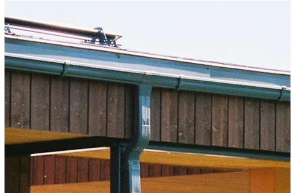
2. K13 gutter and running outlet
