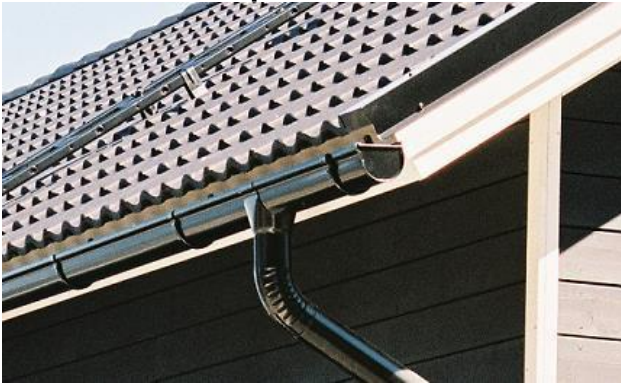
1. P13 gutter with external fixture and running outlet
