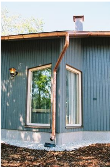
3. P13 copper gutter and 100 mm copper downpipe
