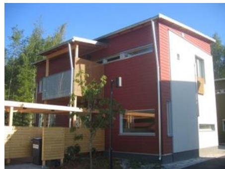
6. 100 mm slanted downpipe
