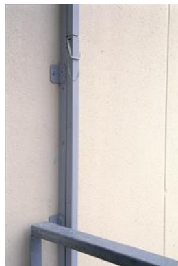
2. Extension of the ladder
