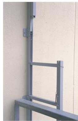
3. Ladder launched at the extension.
